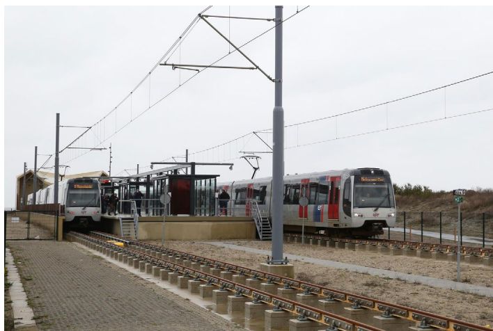
Rotterdam Metro Line B at the new Hoek van Holland Strand station. Maurits van den Toorn photo
