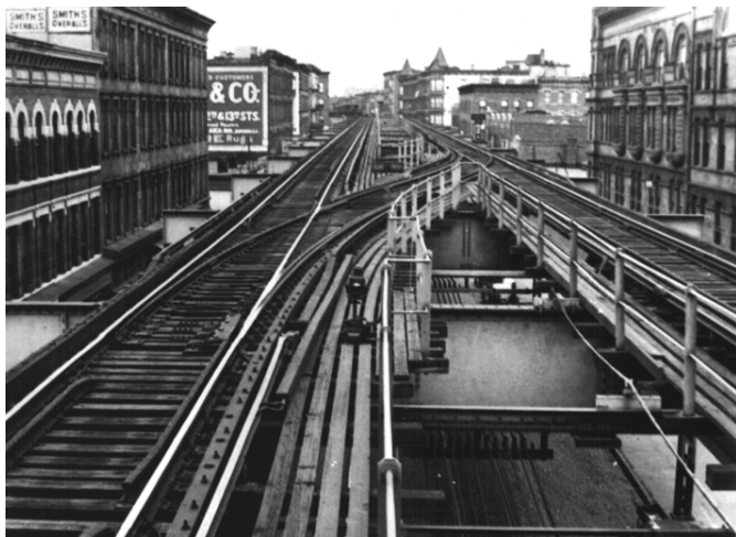
Third Street station looking north — switch in foreground is a hand-thrown switch. Bernard Linder collection
