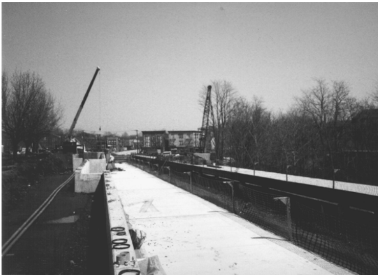
The Bay Street station takes shape.
