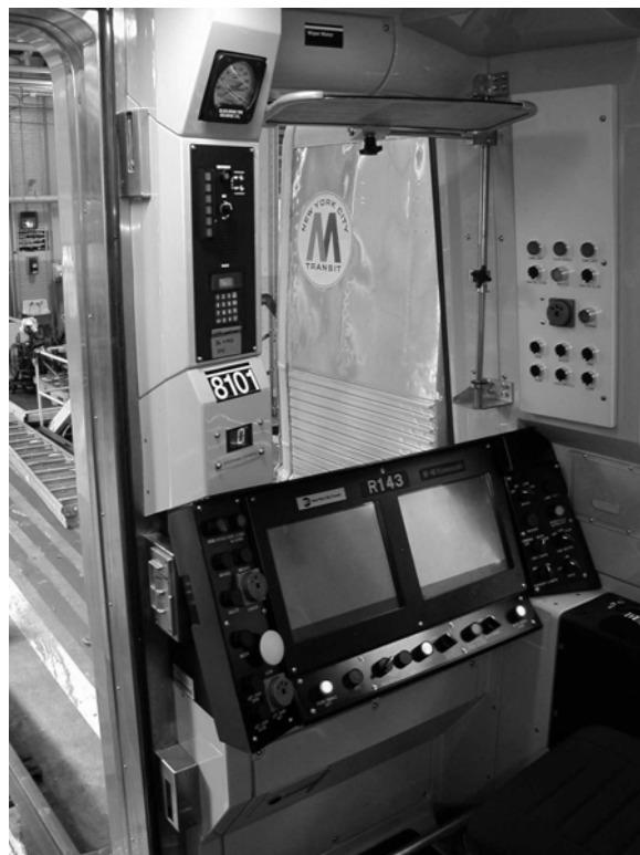
Operating cab of R-143 8101 on May 14, 2001. Note the dual computer screens. Jeffrey Erlitz photograph
