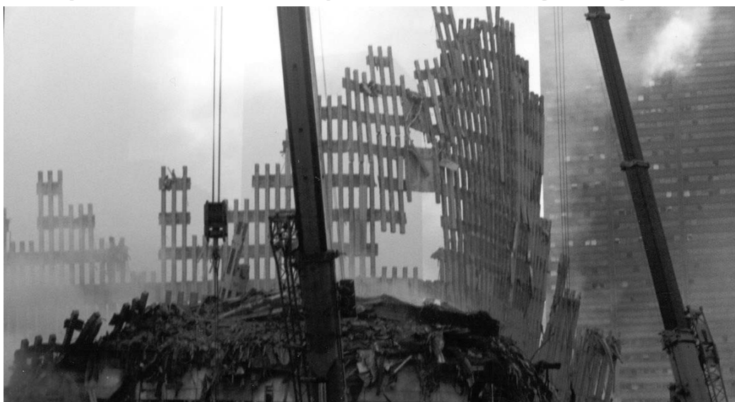
This dramatic photograph, taken on the morning of September 12, 2001, shows the level of damage done to the Twin Towers about 24 hours before.
