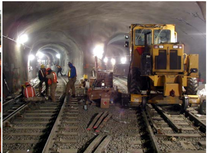
New eastbound crossover west of Exchange Place station, looking east.
