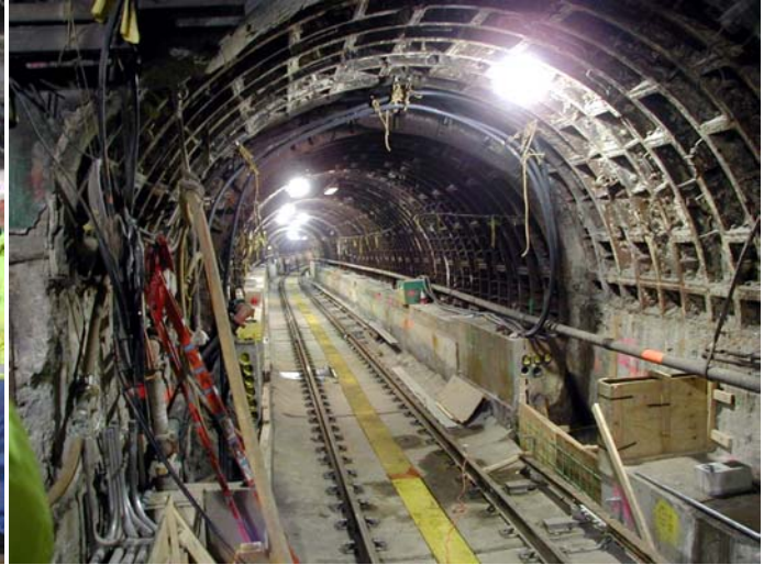
Tunnel F, east of Exchange Place.
