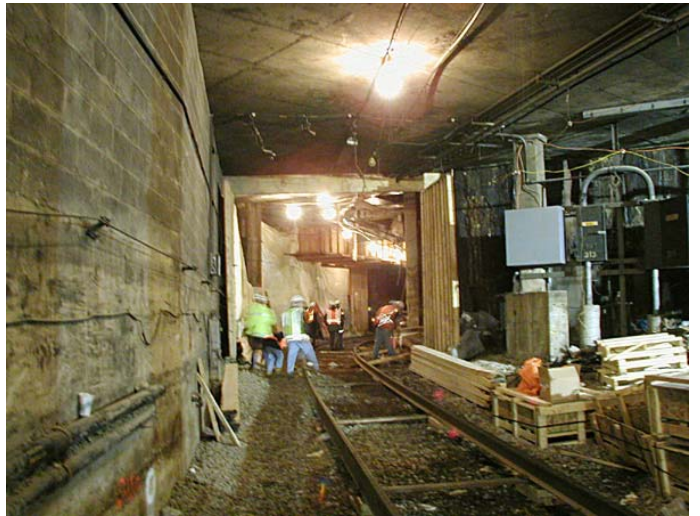
West slurry wall at Tunnel E.
