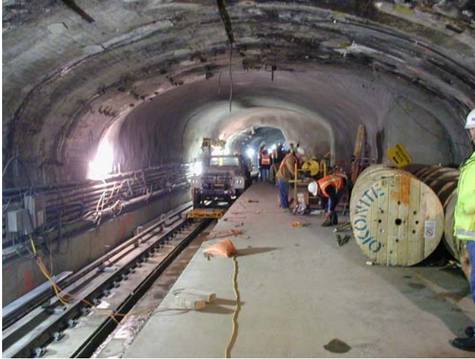
New westward extension of the eastbound platform at Exchange Place.
