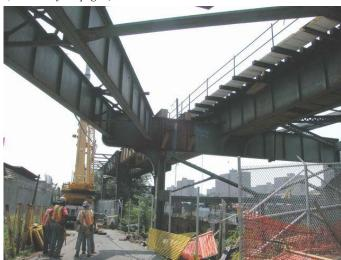
Interestingly, steel shims were installed on top of the northernmost girders of the original structure before the changeover point (see image below) to provide a smooth gradient from the original structure to the new structure. As you can see from one of the images below, several pieces of original Fulton Street El steelwork had already been removed from above former Track P2. This work had been done sometime in the past two years.
