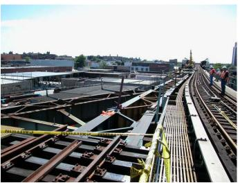
New steelwork for Track Q2 meets the existing portion of Track Q2 north of Sutter Avenue.
