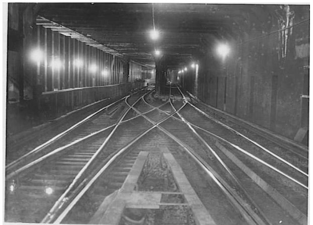
Southbound tracks, looking north, north of the Myrtle Avenue station prior to reconstruction.
