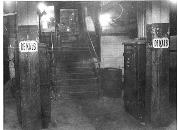
DeKalb Avenue's northbound platform, showing the old tower at the north end. Bernard Linder collection
