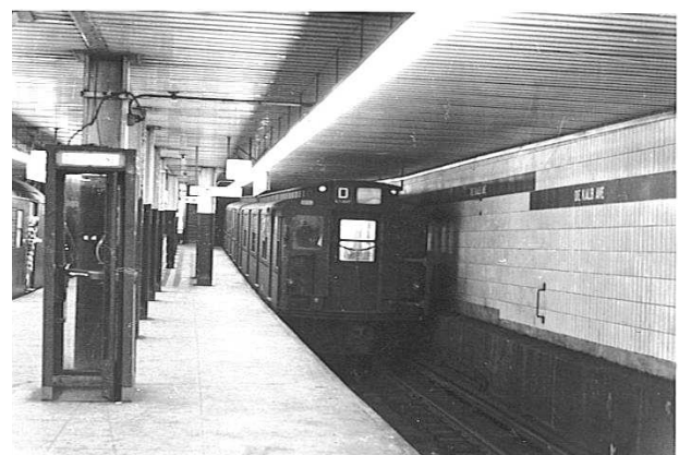
DeKalb Avenue's northbound platform, looking north, February 10, 1969. Note the false ceiling, installed as part of the reconstruction project. Bernard Linder collection
