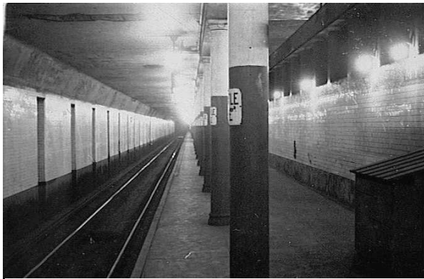
The southbound platform of the Myrtle Avenue station, June 25, 1956. This platform was destroyed in the DeKalb Avenue Reconstruction project of the late 1950s/early 1960s.
