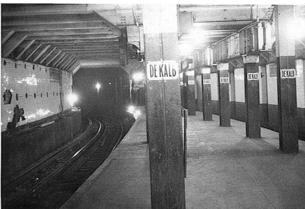
DeKalb Avenue's northbound platform, looking south, October 3, 1956. Bernard Linder photograph
