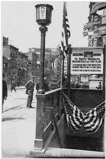
Lawrence Street at Willoughby Street, looking north, at opening of station, June 11, 1924.
