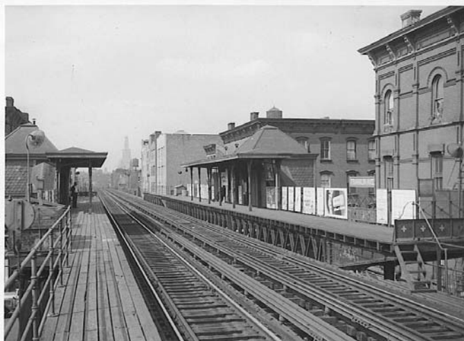
Franklin Avenue station looking west, September 15, 1950. Bernard Linder collection
