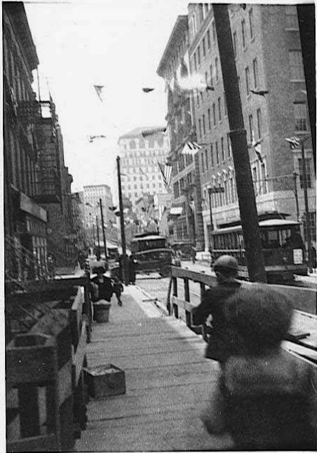
Willoughby Street near Lawrence Street, looking west, during station construction.
