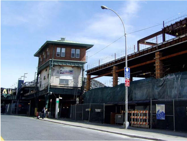
The old tower, on Stillwell Avenue at Mermaid Avenue.
