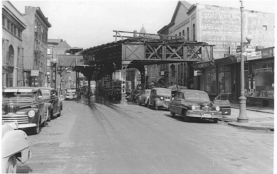
Cables supplying power to the Myrtle Avenue "L" were attached to the Lexington Avenue "L" structure on Grand Avenue between Lexington Avenue and Myrtle Avenue. This structure could not be torn down until a duct line was built. This picture was taken on February 18, 1952 at Grand and Lexington Avenues, looking north. Bernard Linder collection
