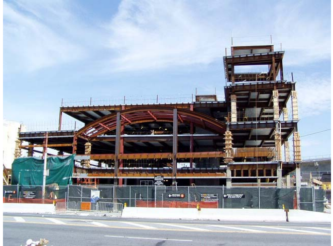
Main entrance, corner of Surf and Stillwell Avenues.
