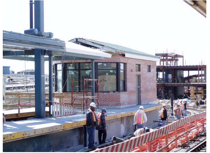
Culver Line Train Dispatcher's office.
