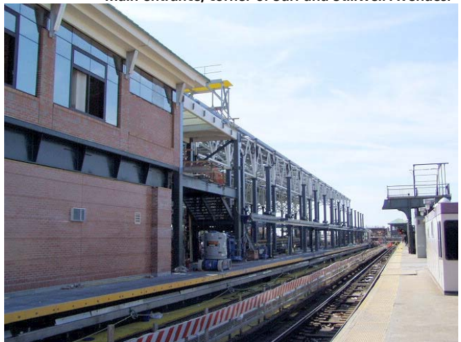
Crew quarters takes shape on the Culver Line (F) platform.
