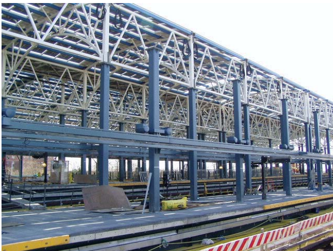
A view of the Culver Line end of the train shed.
