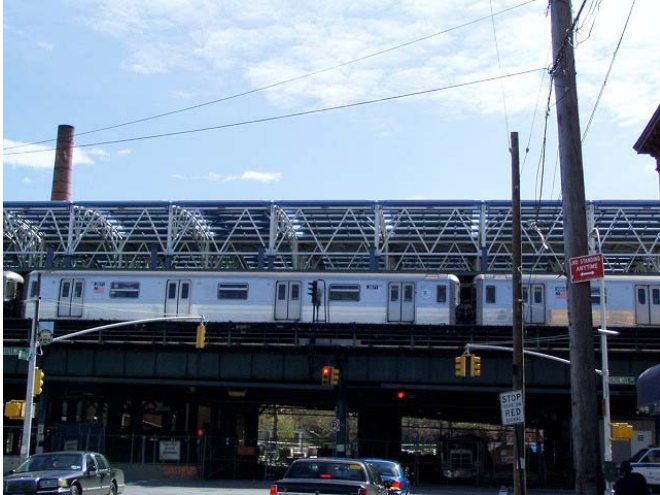
Stillwell Avenue at Mermaid Avenue, looking east.
