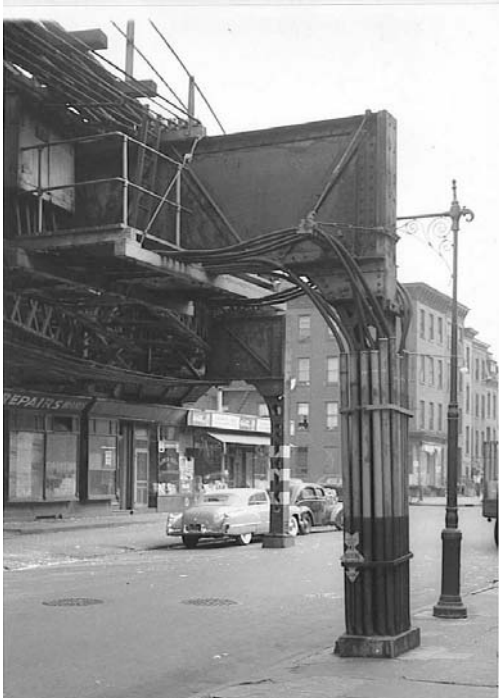
Magnetized column in front of substation at Grand and Lexington Avenues, looking south on Grand Avenue, September 15, 1950. Bernard Linder collection
