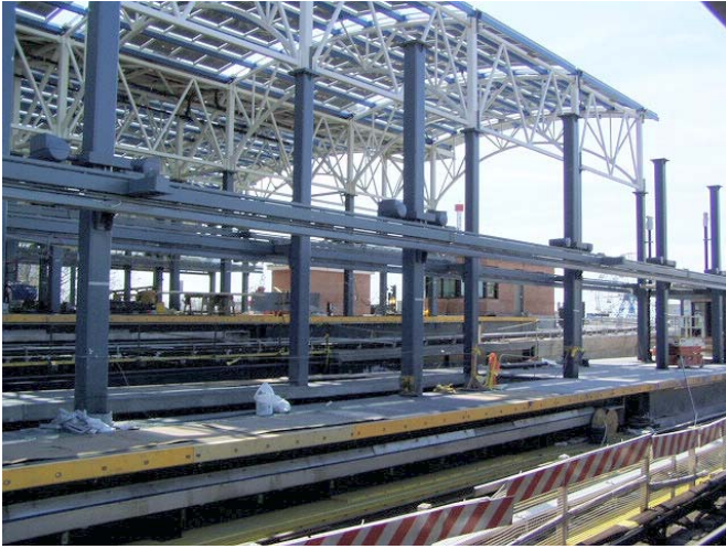
The "front" end (for departing trains) of the Culver Line platform.
