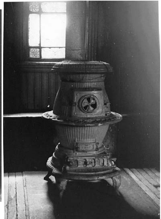
Reid Avenue station, eastbound side waiting room interior. Bernard Linder collection
