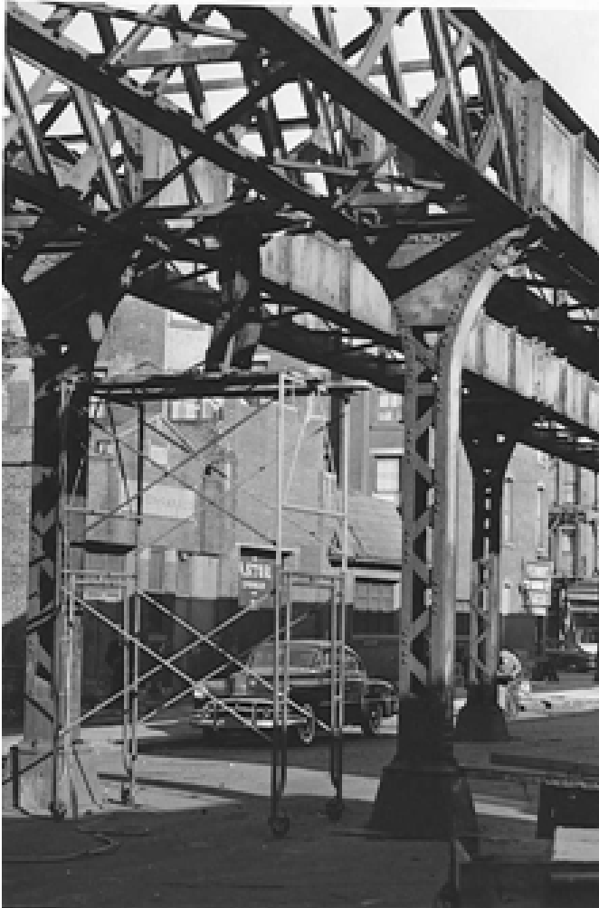
Looking east toward Bedford Avenue.
