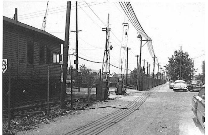
The gates are up, but there is no automobile traffic in this lightly-traveled area (May 25, 1959). Bernard Linder photograph
