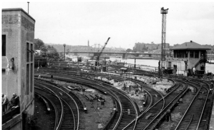
This image of 147 th Street Yard was taken on June 18, 1959. Bernard Linder photograph
