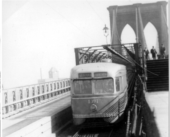
PCC 1091 comes off the bridge.
