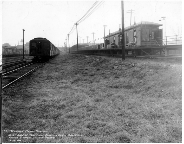
The east side of the platform, tower, and crew quarters, facing south from the layup tracks, also taken on December 9, 1946.
