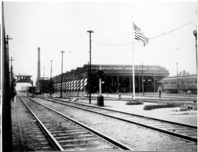
The Fresh Pond elevated shop, shown about 1910. It was later converted to a trolley inspection shop. Bernard Linder collection
