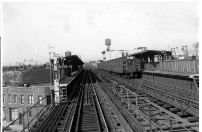
Knickerbocker Avenue station, looking west, April 1, 1969. Larry Linder photograph
