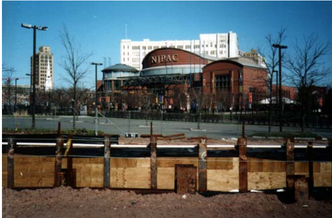
Tunnel portal in front of New Jersey Performing Arts Center.
