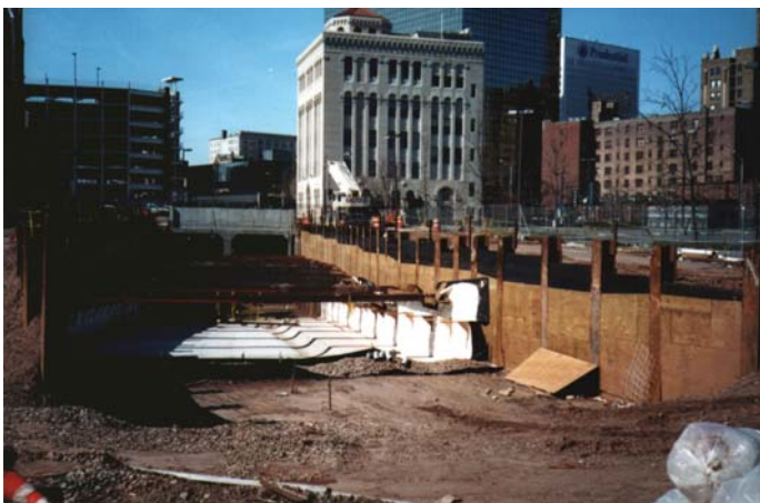
New tunnel portal for extension..
