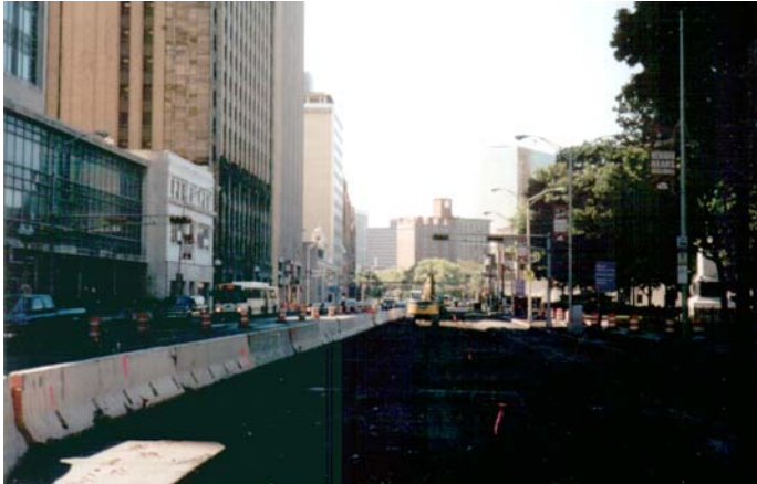
Preliminary excavation on Broad Street.
