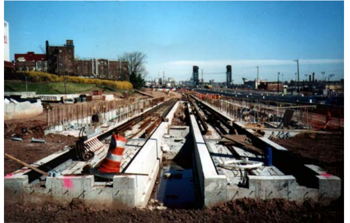
Construction along McCarter Highway.
