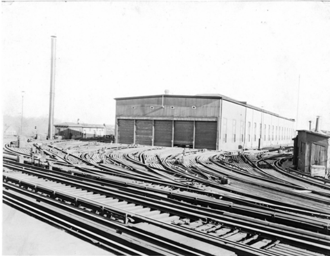
Abandoned inspection shed and yard adjacent to 177 th Street station, December 20, 1924. Bernard Linder collection
