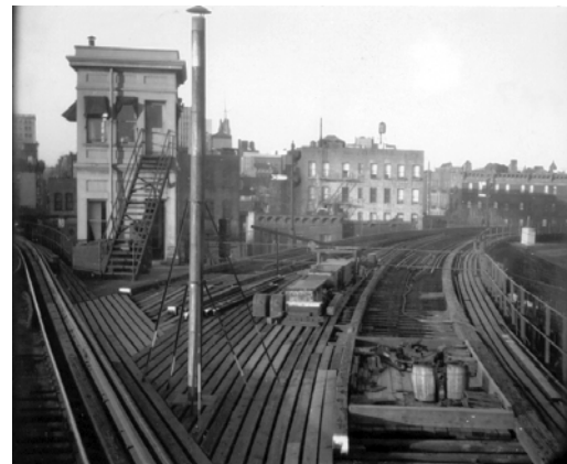
North of the 143 rd Street station of the Third Avenue "L," looking north in 1947, showing abandoned turnouts to the Bergen Avenue Cutoff.
