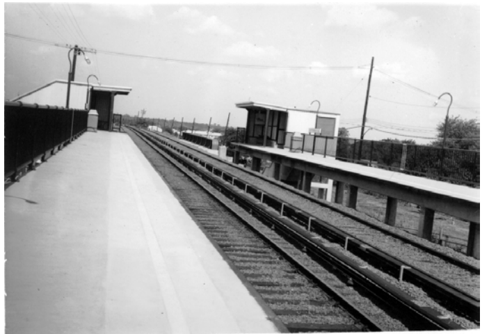
The same scene on August 30, 1968, after grade crossing elimination.
