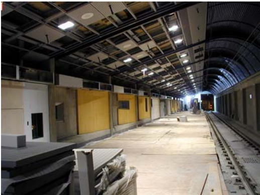
Bergenline station showing northbound (toward Tonnelle Avenue) platform.
