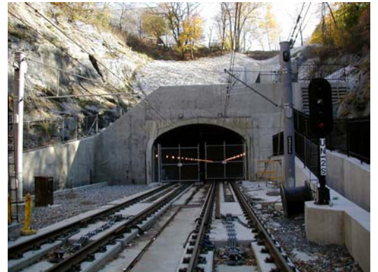
The North Bergen end of the tunnel, with new concrete portal.
