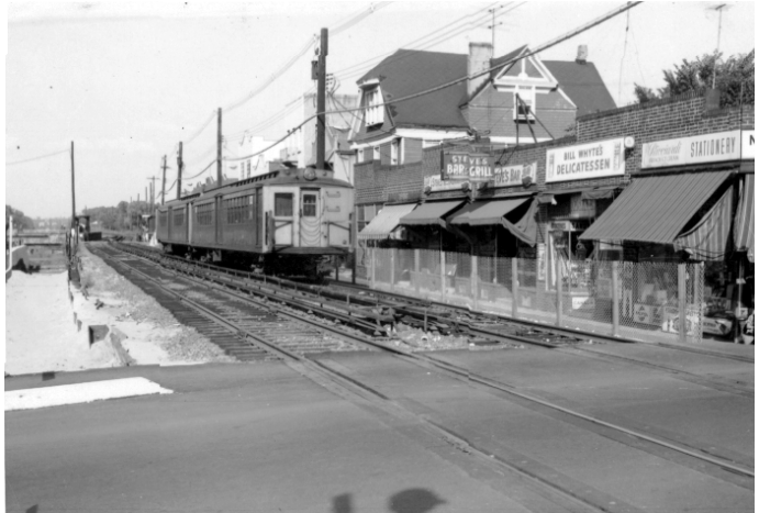
Temporary tracks at Rose Avenue, looking north toward New Dorp station, September 6, 1966. Bernard Linder photograph
