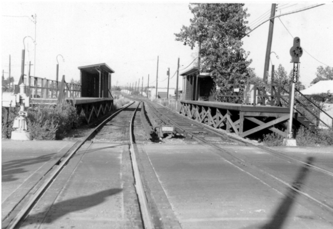
Jefferson Avenue looking north, September 10, 1966, before grade crossing elimination.
