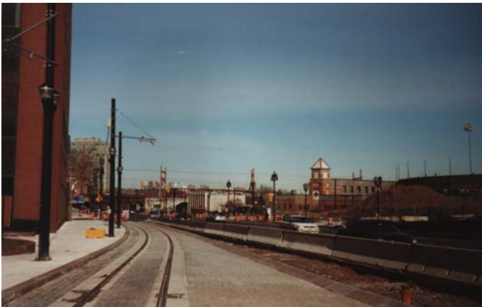
Completed track (southbound) on Broad Street.
