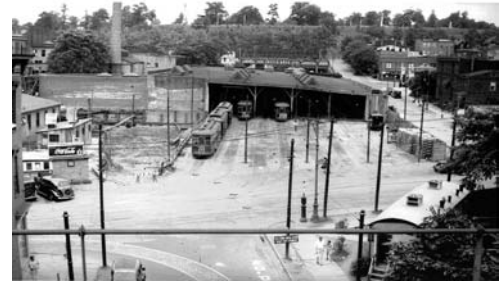
East New York Depot, Jamaica and Georgia Avenues, July 4, 1940.
