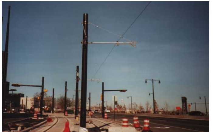
Double-track section parallel to McCarter Highway, Newark.
