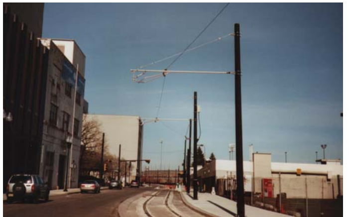
Northbound track is located behind office buildings. Wire now being installed.
