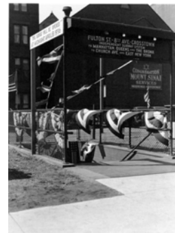
Stairway at Hoyt-Schermerhorn station with banner announcing the opening of the new subway.
