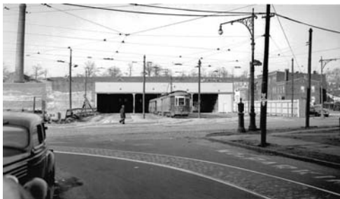
Car 4303 is seen outside the depot on February 9, 1941. The depot was altered to accommodate subway construction.
