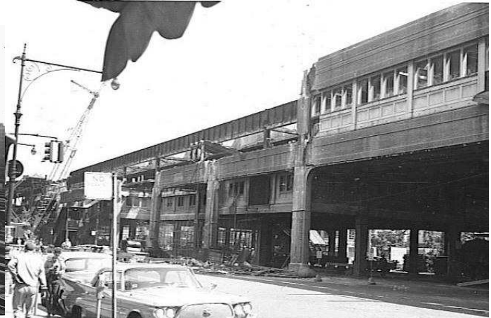
Queensboro Plaza, looking east from street level on June 7, 1962. Bernard Linder photograph
