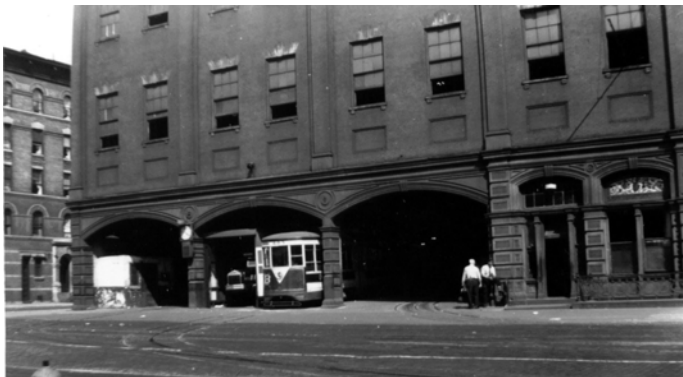
Amsterdam Car House at Amsterdam Avenue and W. 129 th Street, July 28, 1946. Bernard Linder photograph
