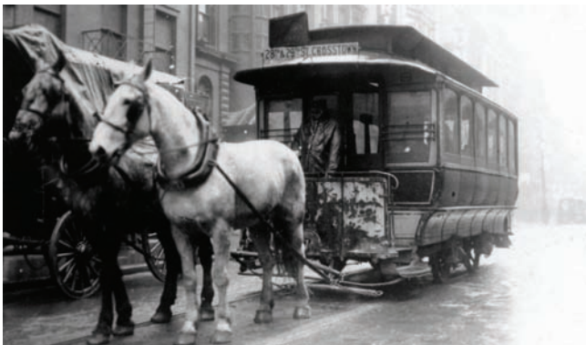
In December, 1910, battery cars replaced the horse cars on the 28 th and 29 th Street Crosstown Line, shown in this March 23, 1908 photo.
