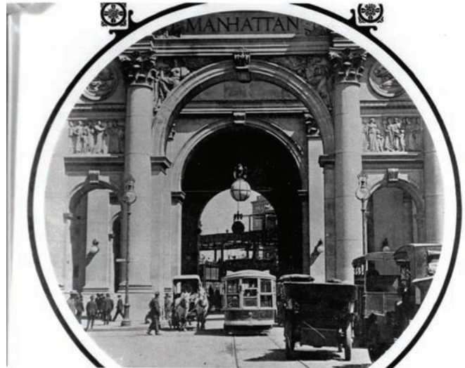
Chambers Street under the Municipal Building in 1915. The IRT City Hall elevated station, which was being rebuilt, is in the background.
