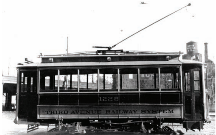
Harlem Shuttle ex-battery car 1228, rewired for 600-volt operation.
