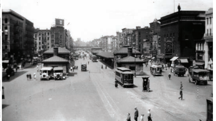
Delancey Street, with storage battery car at the far right.
