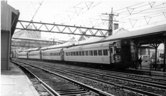
Mount Vernon station, looking south.
