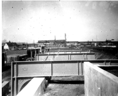
Two photographs of Liberty Junction under construction. Bernard Linder collection
