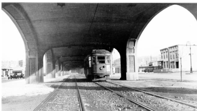
Car 110 is seen under the Flushing Line elevated structure. Bernard Linder collection
