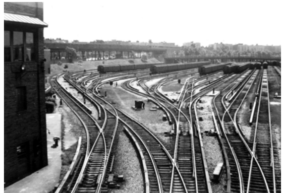
Concourse Yard, looking south from W. 205 th Street, August 31, 1946. Bernard Linder photograph
