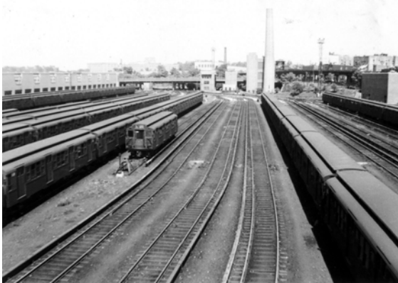
Concourse Yard, looking north from Bedford Park Boulevard Bridge, August 31, 1946. Bernard Linder photograph
