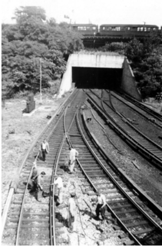
Portal at Concourse Yard, August 31, 1946. Bernard Linder photograph
