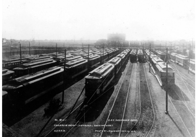
Canarsie Depot's yard, September 12, 1916.
