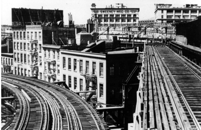
Kings County station, otherwise known as Brooklyn Bridge station, looking north on June 9, 1941. The interlocking was removed from service on January 22, 1934. The curved tracks led to Fulton Ferry. Bernard Linder collection
