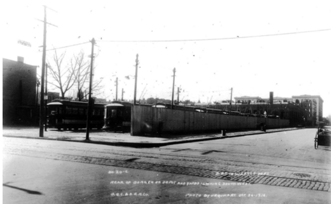
Bergen Street Depot looking southwest, October 26, 1916. Bernard Linder collection
