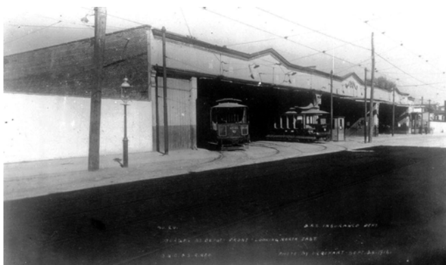
Bergen Street Depot looking northeast, September 26, 1916. Bernard Linder collection
