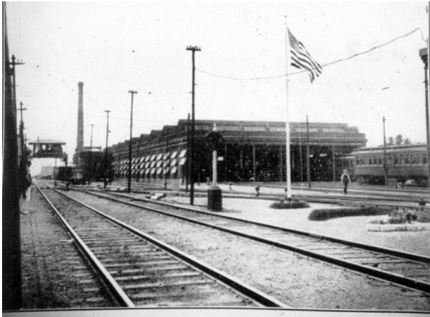
Fresh Pond elevated inspection shop ca. 1910. Bernard Linder collection
