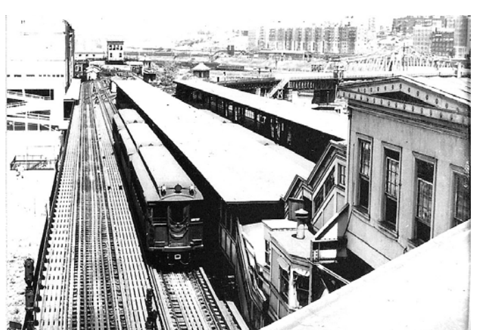
Ninth Avenue Elevated, looking north from 155 th Street. This view was in place until 1940. Bernard Linder collection
