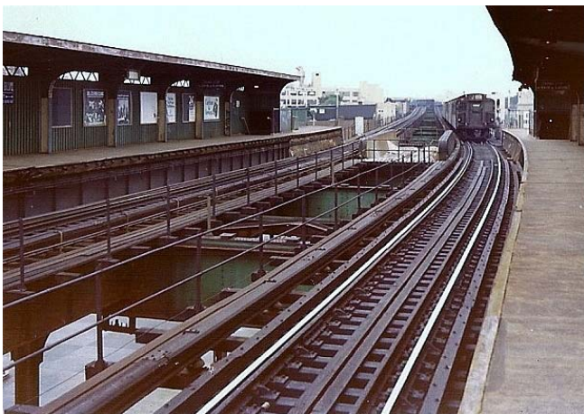
Queens Boulevard station looking west. Bernard Linder collection
