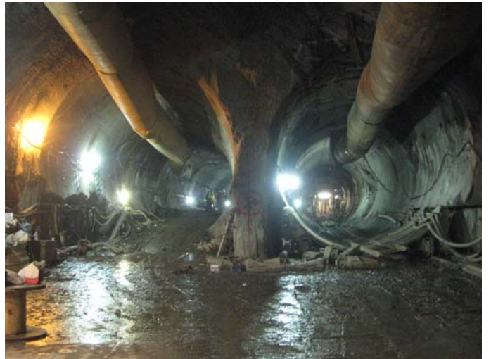
Tubes under construction.
