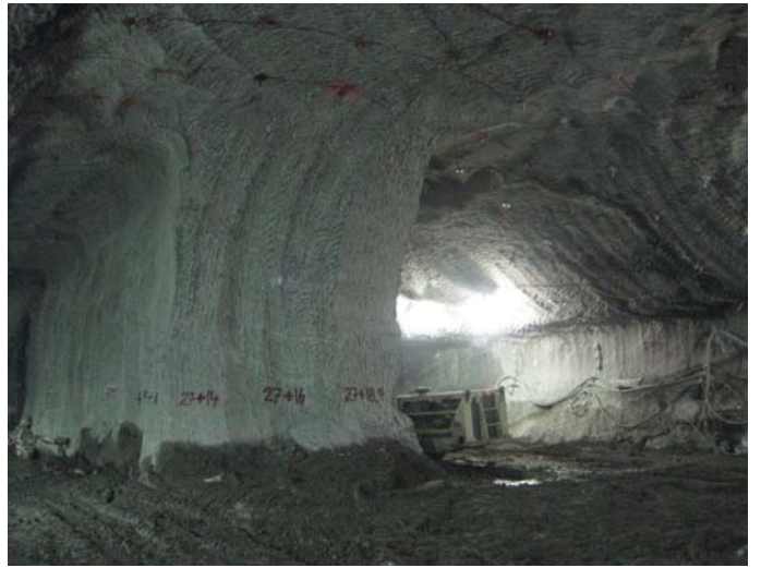
Walls showing results of the Tunnel Boring Machine.
