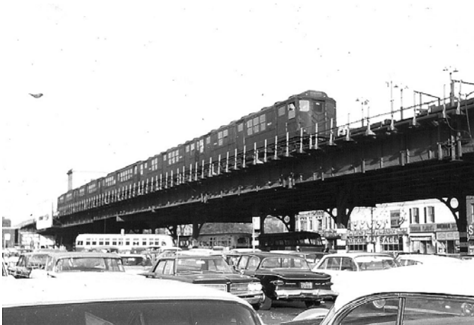
Fordham Road station as seen from street level, November 6, 1965. Bernard Linder photograph
