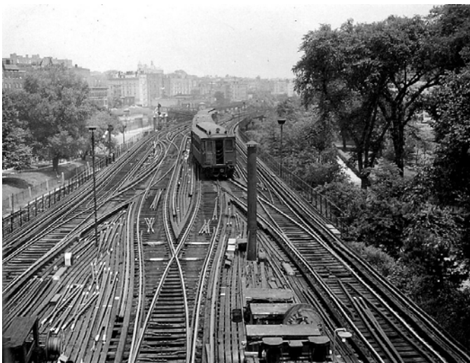
Looking north from the Fordham Road station, June 17, 1951. Bernard Linder collection
