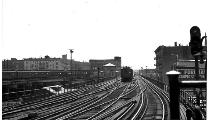
View south from 180 th Street (northbound local approaching), April, 1938.
