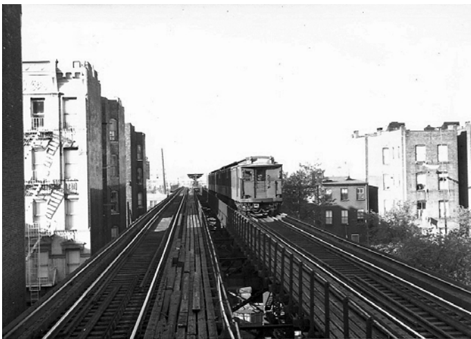
View south from 138th Street, showing backyard section, May 12, 1955. Bernard Linder collection
