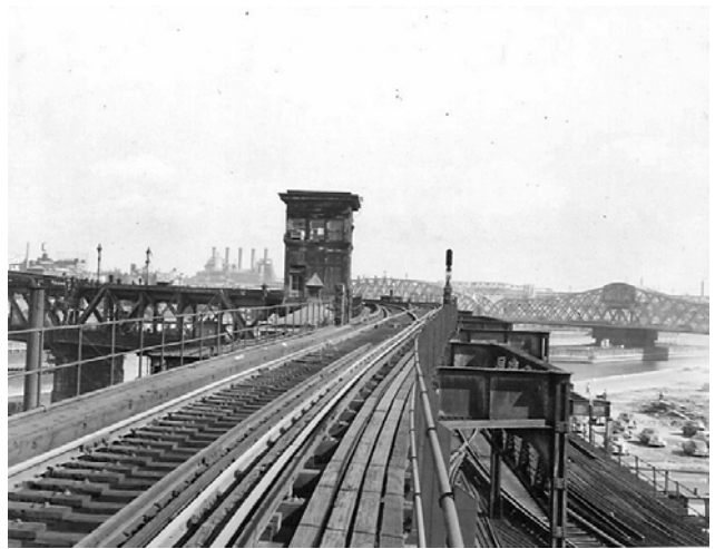
129 th Street station looking east, September 22, 1954. Bernard Linder photograph
