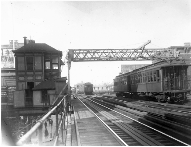
View north from 128 th Street, April 17, 1903 (before third-tracking).
