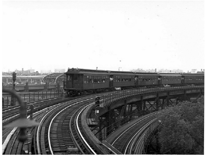
Thru express gate train south of 133rd Street, July 8, 1950. Bernard Linder collection
