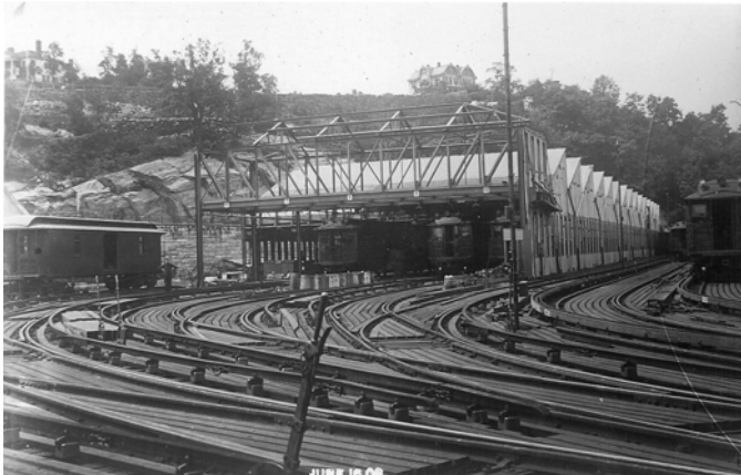
Inspection shed under construction in June, 1903.
