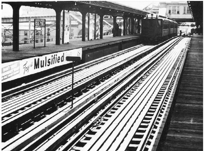
155 th Street-Eighth Avenue station looking south.
