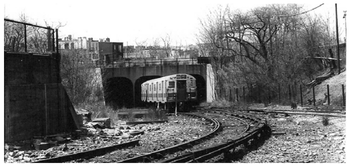
Portal east of Ninth Avenue station looking west, April 23, 1975. Bernard Linder photograph
