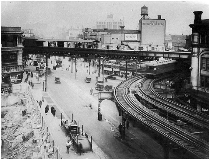
Fifth Avenue El crossing under Fulton Street El east of Flatbush Avenue, 1927. Bernard Linder collection
