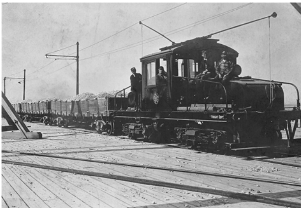
South Brooklyn Railway engine 5 leaves the 63 rd Street dock with a draft of cars loaded with broken stone to be used in connection with the rebuilding of the Brighton Line.
