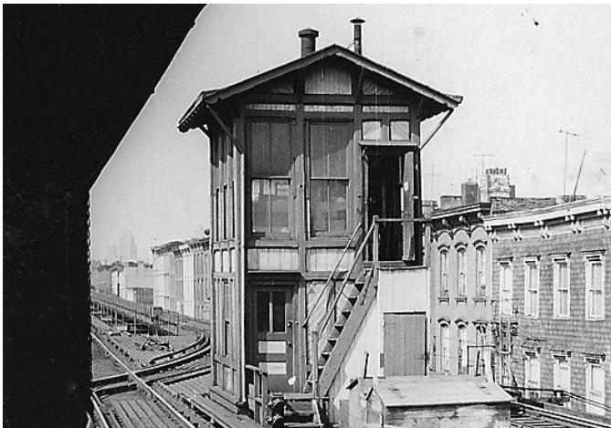
Tower at Myrtle and Grand Avenues, Lexington Avenue Elevated, September 15, 1950. Bernard Linder collection
