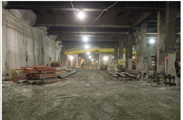
Tracks removed, beams removed.
