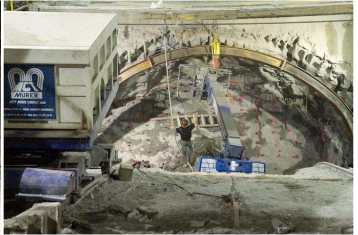
Construction worker shows the project's size.
