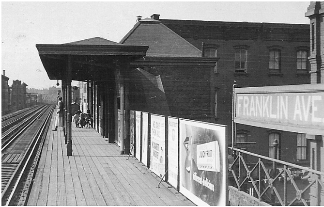
Franklin Avenue station, Lexington Avenue Elevated, looking west, October 5, 1950. Bernard Linder collection
