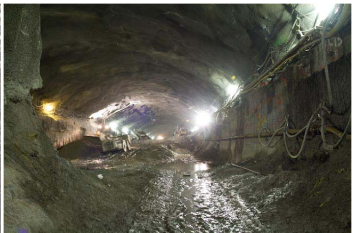
A 300-level tunnel south of E. 48th Street.
