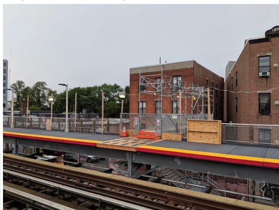
Temporary staircase from the north side of Atlantic Avenue between Nostrand and New York Avenues to the westbound platform. The fiber-reinforced polymer platform can be seen here.
