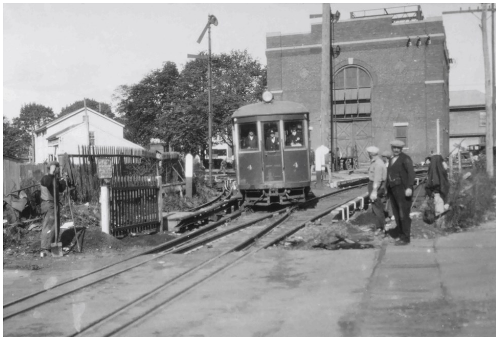
Battery car 4 is on the west leg of the wye at Mineola in September, 1926. The third rails are newly installed and will be placed into service the following month. With that, the battery cars will no longer be used on the branch. Substation #8 is in the background, along with MT (now Nassau) Tower to the right of it. Both of those structures are still standing today, but will be demolished very soon.
