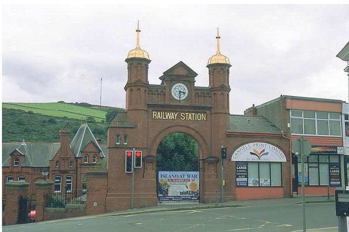
(Above and Below) The red brick used to build the Isle of Man Railway passenger station in Douglas evokes an impression of Britain's industrial era. The buildings were constructed between 1887 and 1913 of Ruabon brick, fabricated from clay in Wales and used throughout the British Isles. The upper view shows the grand archway, the original main entrance to the terminal, topped with two gilt turrets and a clock tower. The gates were closed, and we walked down a hill to the vehicle entrance, where we found the bus shown below. The conveyance was built by Thornycraft in 1928 for the Isle of Man Railway, when the company began to supplement its rail services with road transport. The building in the background houses the railway's ticket office and The Tickethall restaurant, as well as tourist information and a waiting room.
