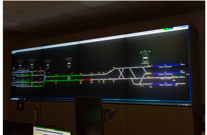
The main display screen in Grand Central’s Train Operations Center (TOC) on January 6. The white track segments have no route established through them, green indicates an established route, red is an occupied block and the blue segments have “holds” on them, meaning a train is not allowed to enter them. A hold would be the same as to a “lever blocking device” on a mechanical interlocking machine.
