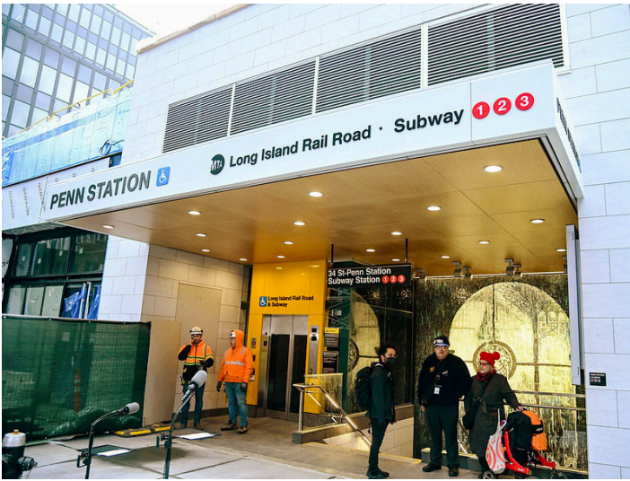
View north of the new 34th Street-Seventh Avenue entrance.
