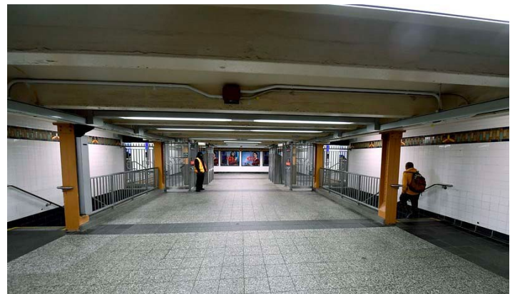
Looking west at the expanded mezzanine at Main Street on November 22. Marc A. Hermann/MTA photo
