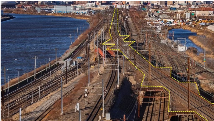
Looking west at the Sawtooth Bridges in Kearny. Amtrak photo
