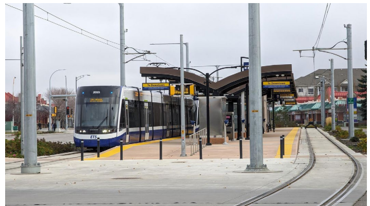
View east of the new Mill Woods terminal at the south end of the line with Bombardier Flexity 2025. City of Edmonton photo
