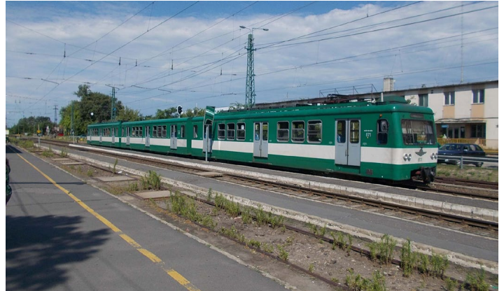
Akin to an S-Bahn, Budapest's "local railway" is the HÉV. In this June 2019 view of EMU 871 (LEW Lokomotivbau-Elektrotechnische Werke, 1971) at the Szigetszentmiklós-Gyártelep stop of the H6 route that runs south to Ráckeve from the Közvágóhíd terminal in Budapest.
