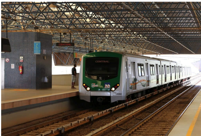
An Alstom Metropolis unit at the current Orange Line western terminal at Samambaia. IRJ photo
