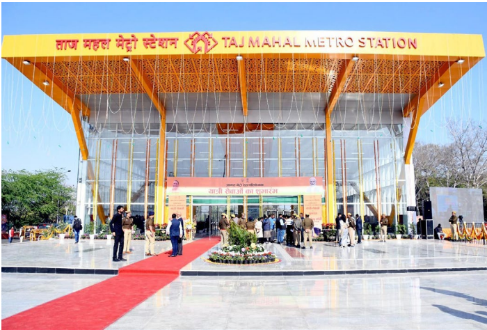
Taj Mahal metro station opening. UPMRC photo
