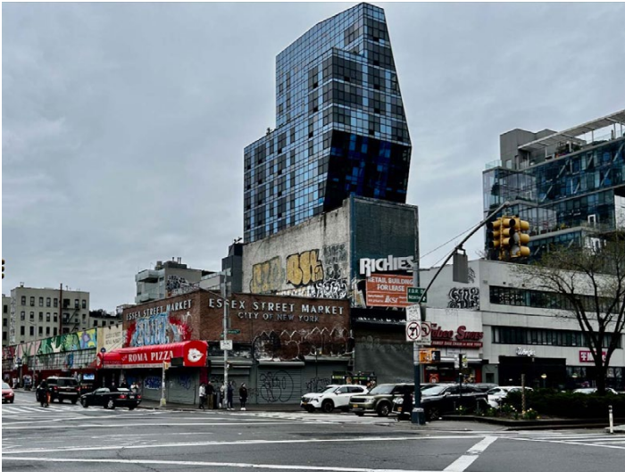
A current view of the northeast corner of Delancey and Essex, formerly the location of the Essex Street Market. This is Site 9 of the Essex Crossing redevelopment project. Lo-Down Productions LLC photo
