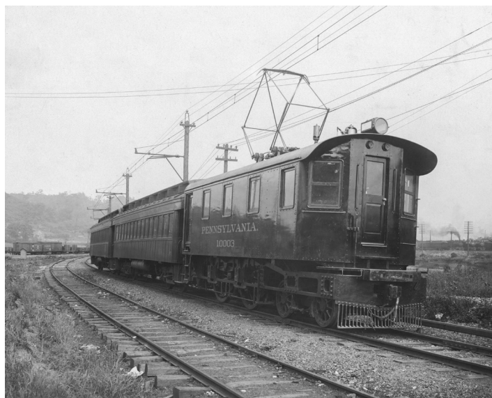
(Above left and right and below) Single-Phase alternating current electric prototype locomotive No. 10003, with two Pennsylvania Railroad coaches (No. 3018 and unknown No.), comprising a demonstration train. Note the brass air whistle following steam locomotive practice, and a carbody designed for high platform access. Location is likely the 1¼-mile electrified test track at the Westinghouse East Pittsburgh works at a press event unveiling the “black monster” in 1907. Pennsylvania Railroad company photograph.
