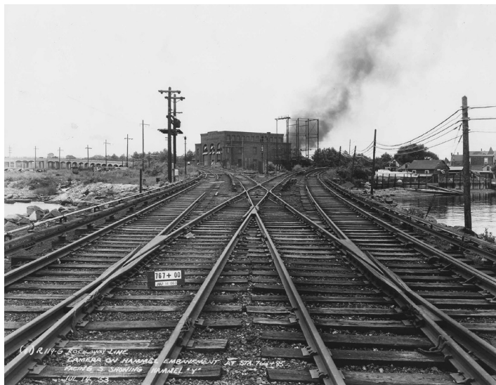
View looking south of the former LIRR at-grade junction at the north end of Hammels Wye on July 14, 1953, about the time reconstruction work for subway operation started in earnest. This view was probably taken by the general contractor to show existing conditions before construction started. Subway Construction Photographs collection, New York Transit Museum
