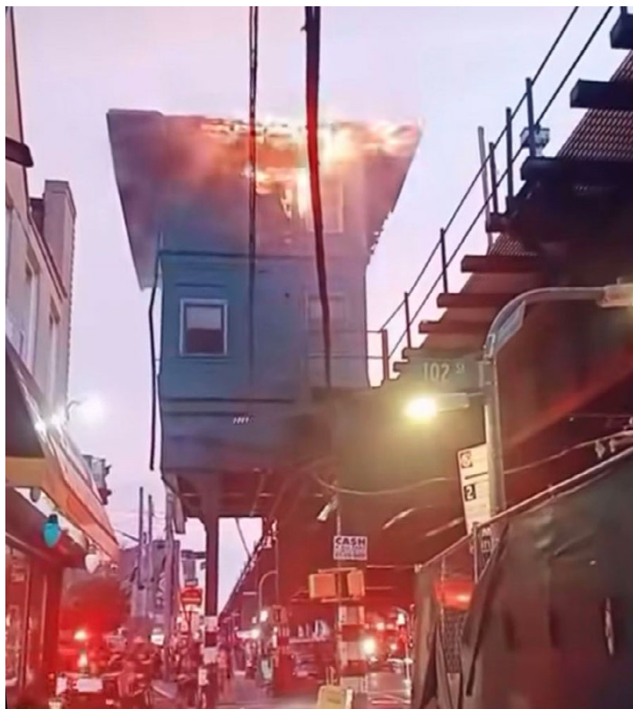
View of the fire from street level, on Roosevelt Avenue and 102nd Street. Unattributed Facebook post photo
