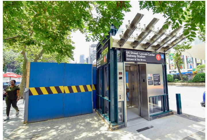
The new elevator from the northbound platform to the street at 66 Street-Lincoln Center. Marc A. Hermann/MTA photo
