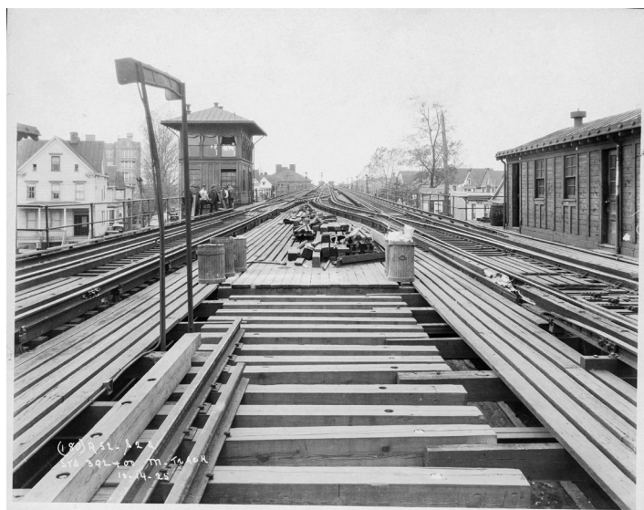
View west from the south (geographically west) end of 103 Street–Corona Plaza Station on October 14, 1925, one day after the line was extended one stop to 111 Street. The interlocking is still, apparently, in service on this day. It could be that trains operated between these two stations on two separate “single-track” operations.
