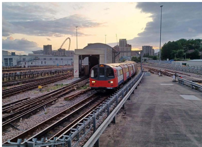
London Underground Neasden depot. Hitachi Rail photo
