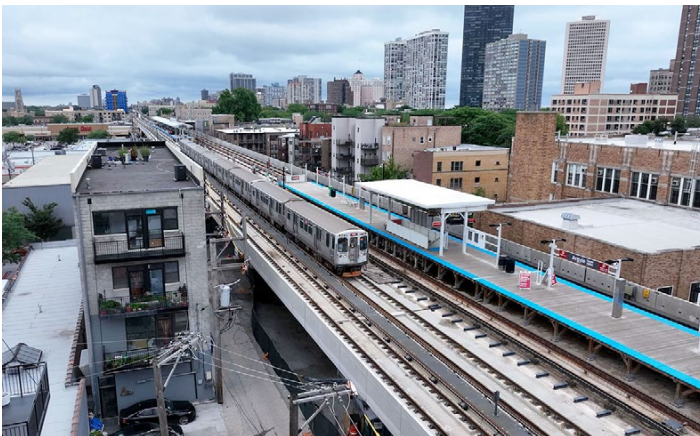
Aerial view of the newly-opened Argyle Station. Walsh-Fluor Design-Build Team photo
