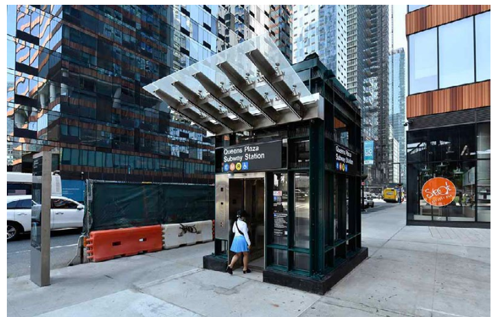
View southwest of the new mezzanine-to-street level elevator, on the corner of Queens Plaza South and Jackson Avenue.
