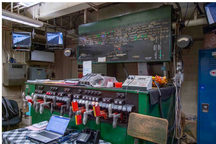
The GRS 32-lever Model 5 machine at 42 Street North Tower on May 24, 2023. Jeff Erlitz photo
