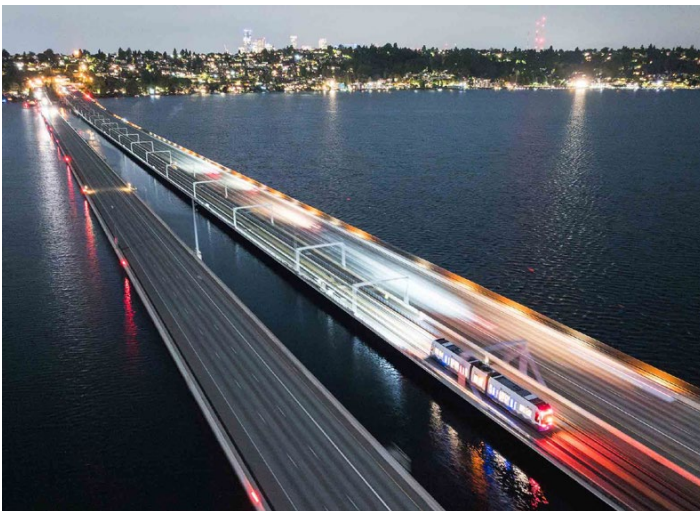
The first run of a powered LRV over the I-90 bridge, on September 8. Peter Bohler/Sound Transit photo
