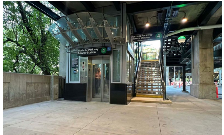
One of the new elevators at Mosholu Parkway, at street level.
