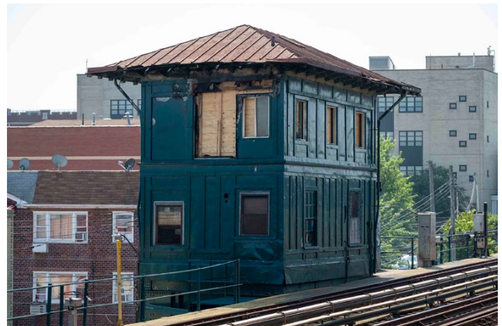
The former Albutis Avenue Tower, as seen on Sunday, August 3, a little over one week after the fire. Jeff Erlitz photo
