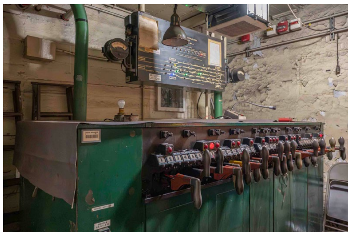
The 40-lever GRS Model 5 interlocking machine at 30th Street Tower on October 21. Jeff Erlitz photo
